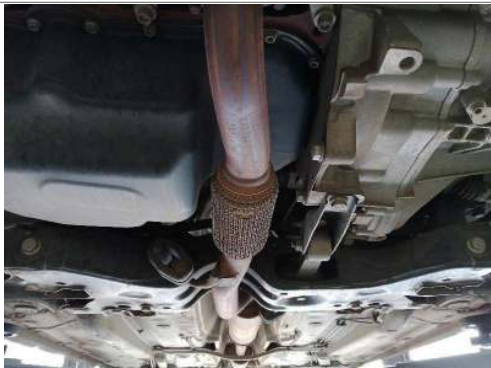
Engine to silencer pipe
