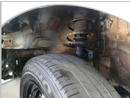
L/F fender liner missing
