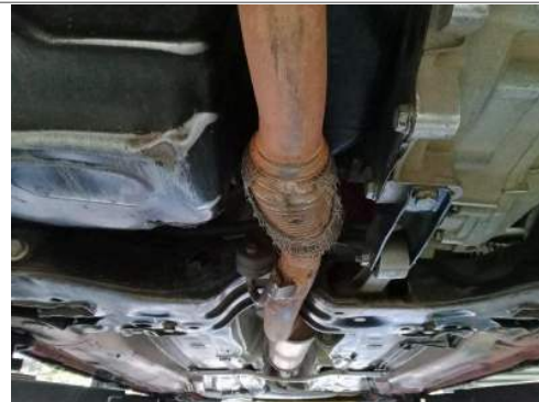
Engine to silencer pipe
