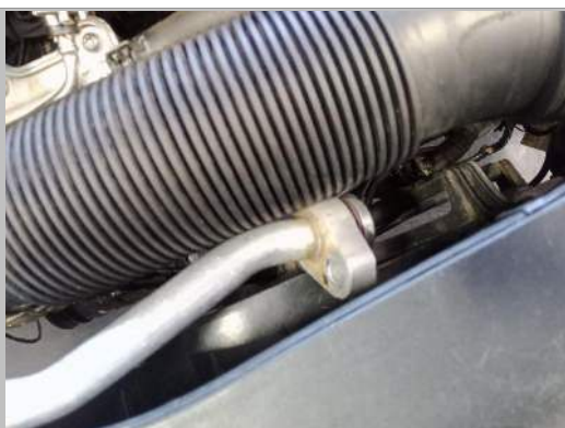
Air conditioner pipes
