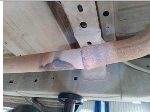
Engine to silencer pipe
