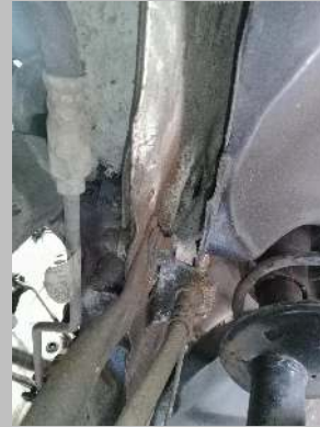
Main Beam Left
