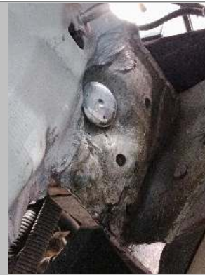
Main Beam Left
