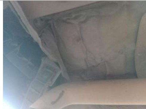
Sparewheel well damage
