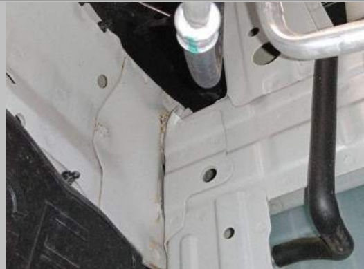
Main Beam Right
