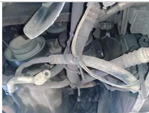
Air conditioner pipes
