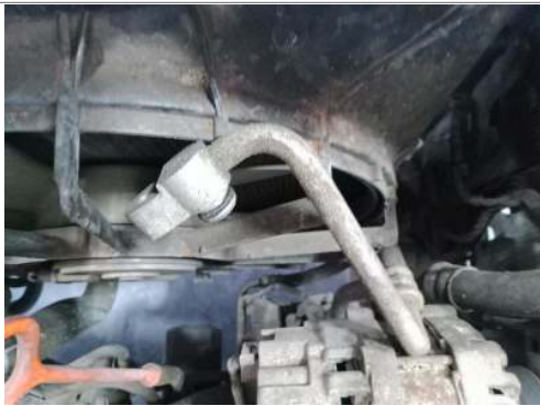
Air conditioner pipes
