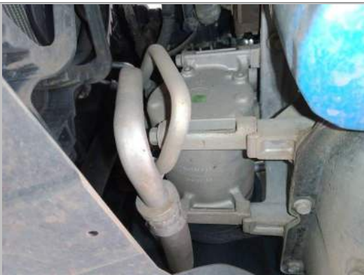
Air conditioner pipes
