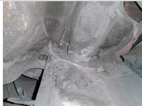
Main Beam Left
