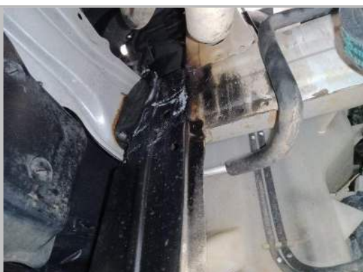
Main Beam Right
