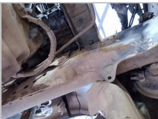
Main Beam Left
