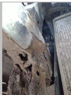
Main Beam Left
