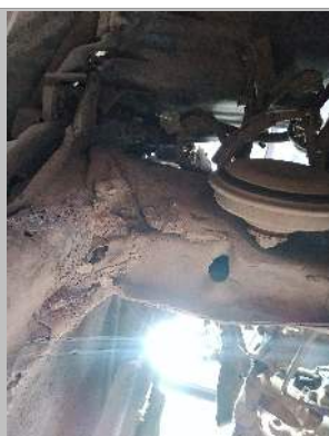
Main Beam Left
