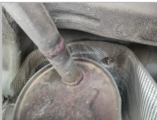
Engine to silencer pipe
