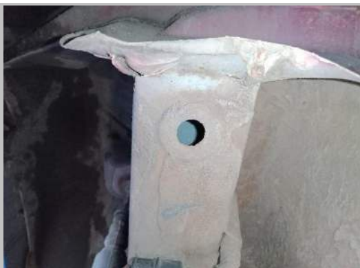
Main Beam Left
