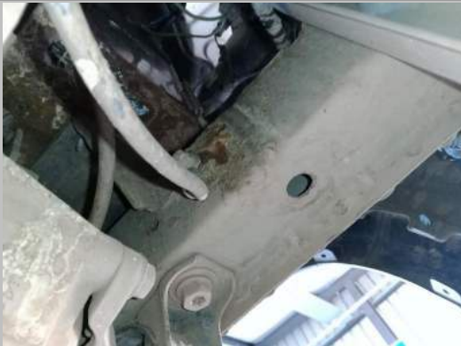
Main Beam Left
