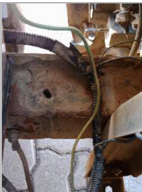
Main Beam Left
