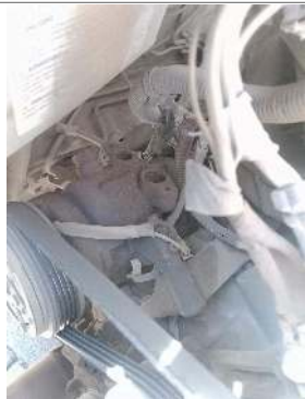
Air conditioner pipes
