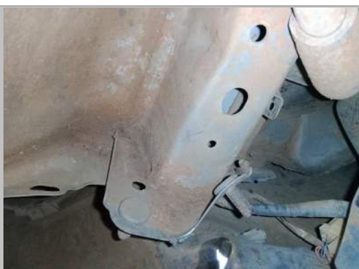
Main Beam Left
