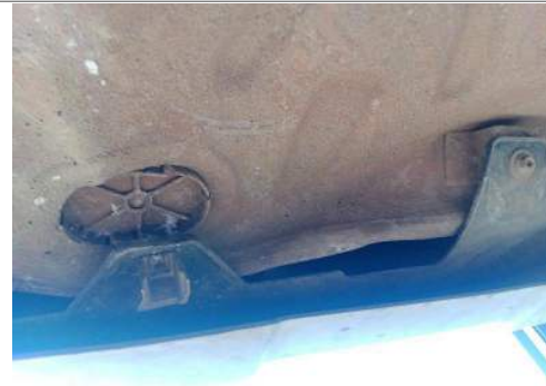
Sparewheel well damage
